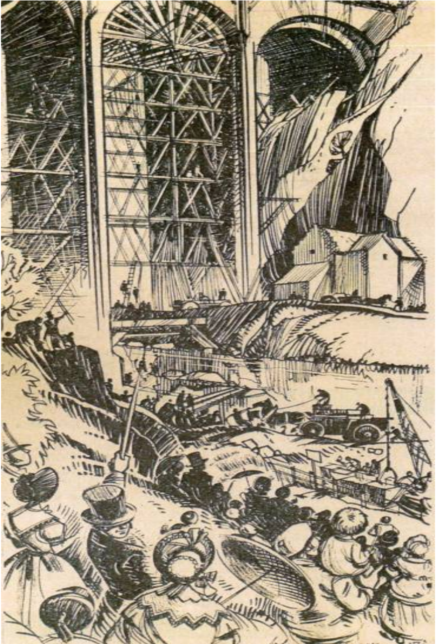
Spectators come to view the building of Dean Bridge (2) (Copyright: reproduced by permission of The Scotsman Newspapers)
