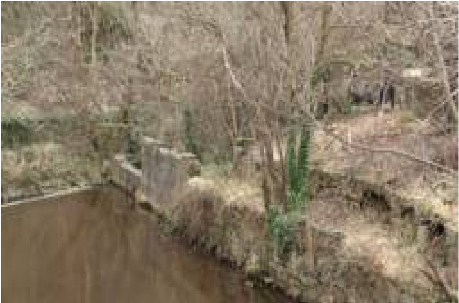
Area on the South side of the lower weir by West Mill below which the hydro-electric generator could be positioned.
